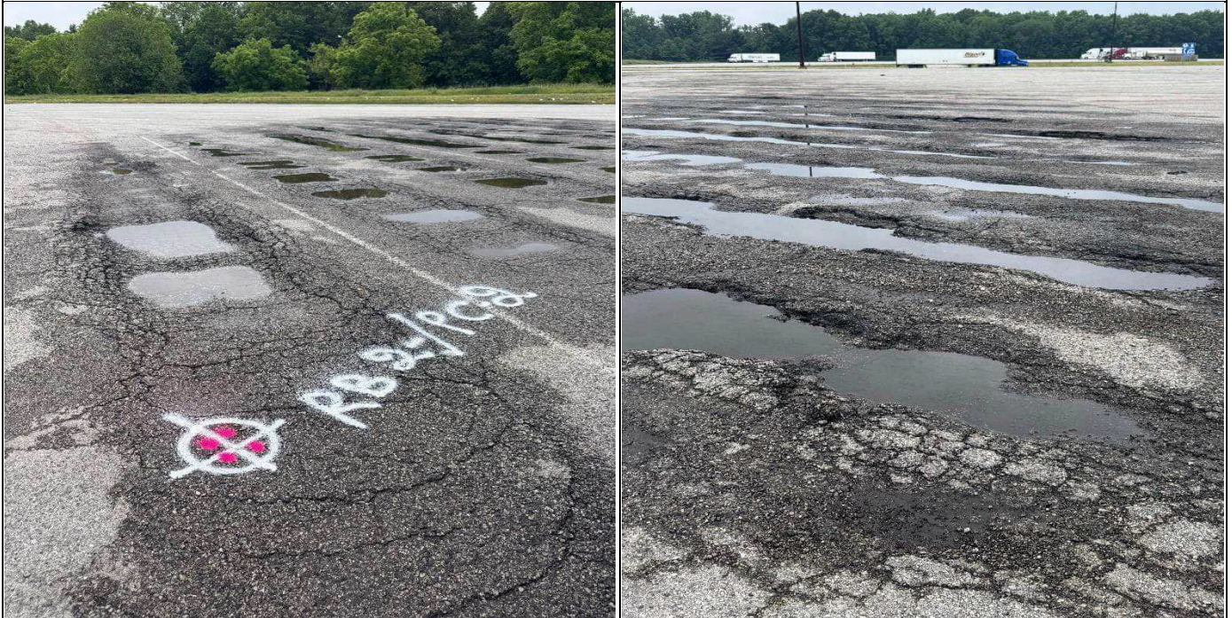
Photographs showing high severity rutting in the parking stalls. We recommended HMA Patching, Full-Depth to fix these and similar distresses.
