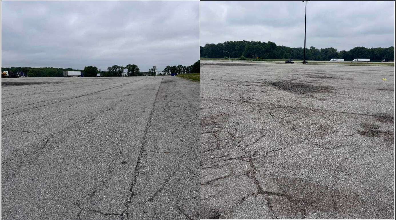
Photographs showing the typical pavement surface condition of the parking lot.
